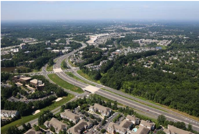
The interchange is in a highly urbanized area of Fairfax County and required close coordination with the public as well as local elected officials.
